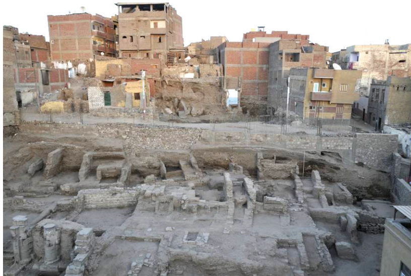
Fig. 16: Area 3: Overview of the eastern section of Area 3 before the construction of the retaining wall.
